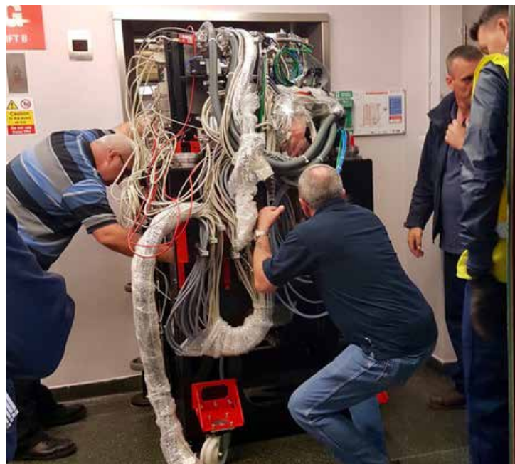
Supplier FEI and Birkbeck's Estates team worked together to manage delivery, including stripping back the lift shaft to accommodate parts of the microscope.
